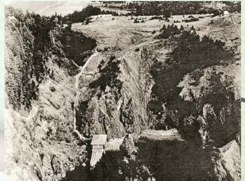
Aerial view of boathouse in Nellies Cove.
